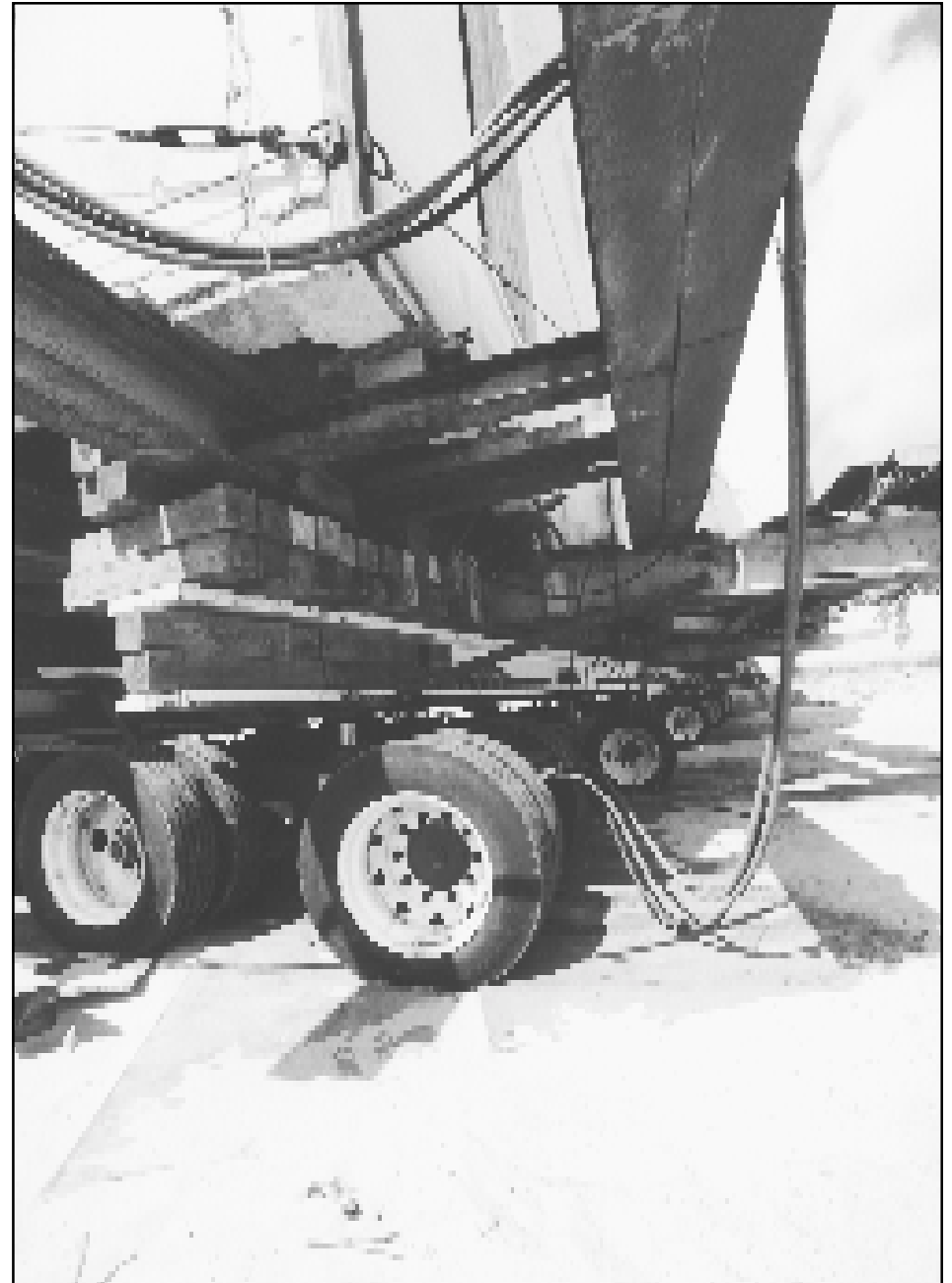
▲ The power for the move is provided by the engine and hydraulic pump, with Phil in control with the remote control on a thirty-foot cable.
